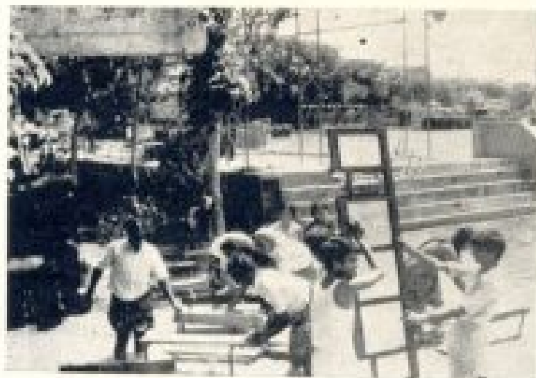
23. Flooding out dust and dirt !
